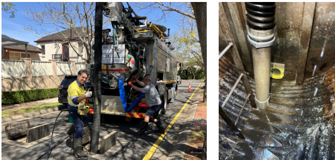
Vacuum truck and interior of one of the 6 underground detention tanks
